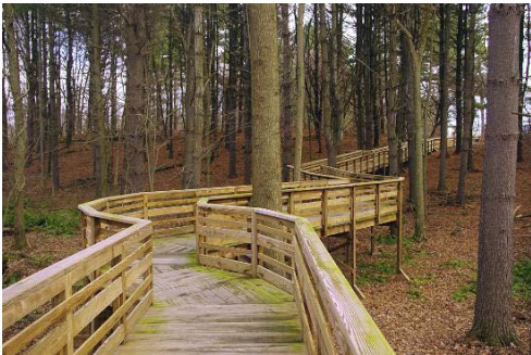
The Silvio Conte trail in Hadley, MA uses wooden footers for their universally accessible boardwalk.
