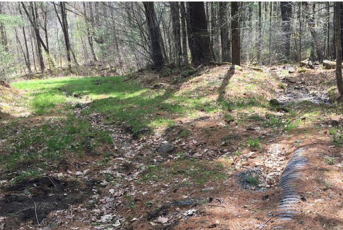
B) Lesser-used roads are muddy with broken culverts.
